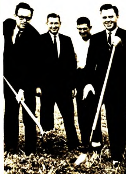
TEXAS CHURCH—Ground is broken by Pastor Homer Butler (left) and Church Trustee Eldon Myler for a $58,000 church at McAllen, Texas. The building will seat 250 persons. Richard Bartholomew (second from left) and Phil Dial, both of the architect's office, watch the ground-breaking. The church is on the San Antonio District.
