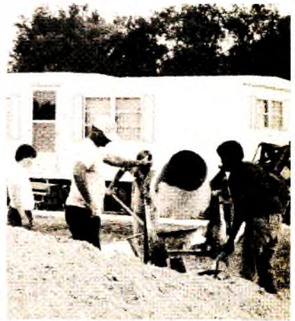
Men mixing concrete for the sidewalks
