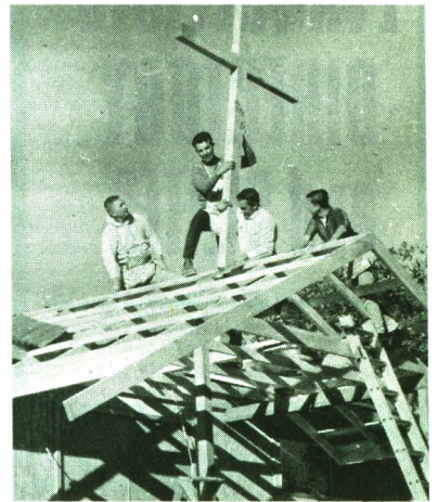
Workers lift the cross onto the new church structure.
