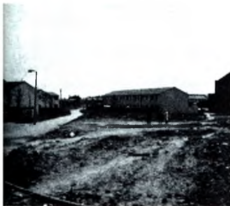
Site of future church on Derbyshire St. in Leeds, England. Construction commenced July, 1976.
